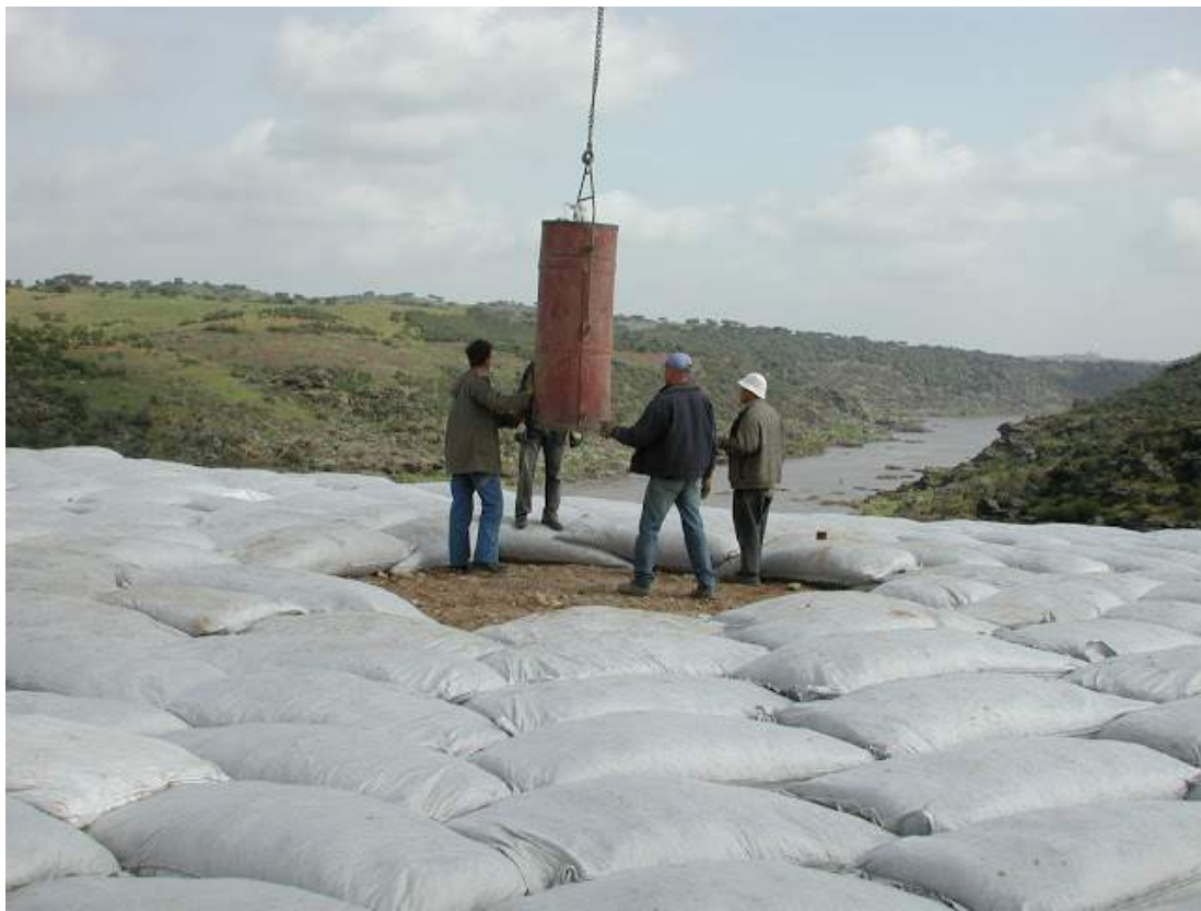
25. Engineers finishing the protective coat for the Louisa castle before its submersion. Photo taken from the Internet.
