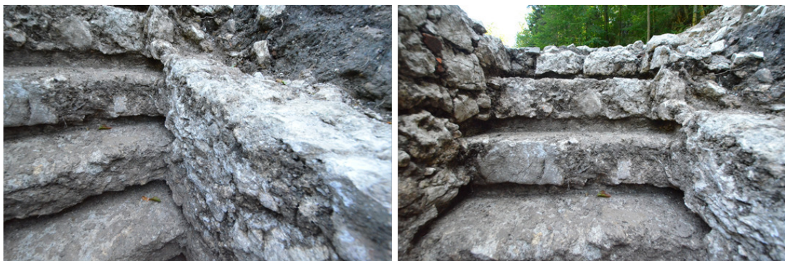
Fig. 6.6: Stairs with recesses for wooden covers in Cellar 2.
