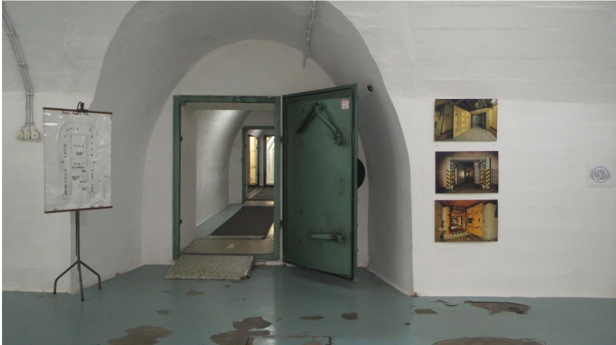
Fig.48. Entrance of block 7, three metal doors to decontamination room, view from the tunnel.
