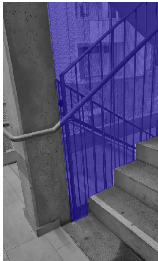
Picture 8 : perforated metallic staircase wall - HAK
