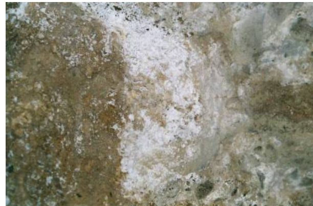
Figure 20 A Picture showing the location and ground plan of St.Virgil; B Red wheeled cross painted onto white plaster; C Salt efflorescence on the stone work of the chapel
