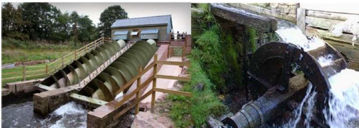
Figure 26: Archimedean screw and impeller 15
