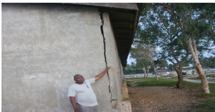
Figure 5.4: One of the heavily cracked school blocks at Adina
