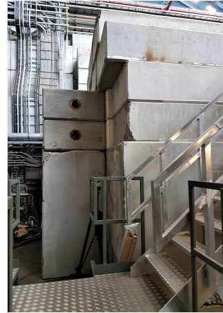
(b) Outside view of the concrete bunker surrounding the setup at PSI for radiation safety.
